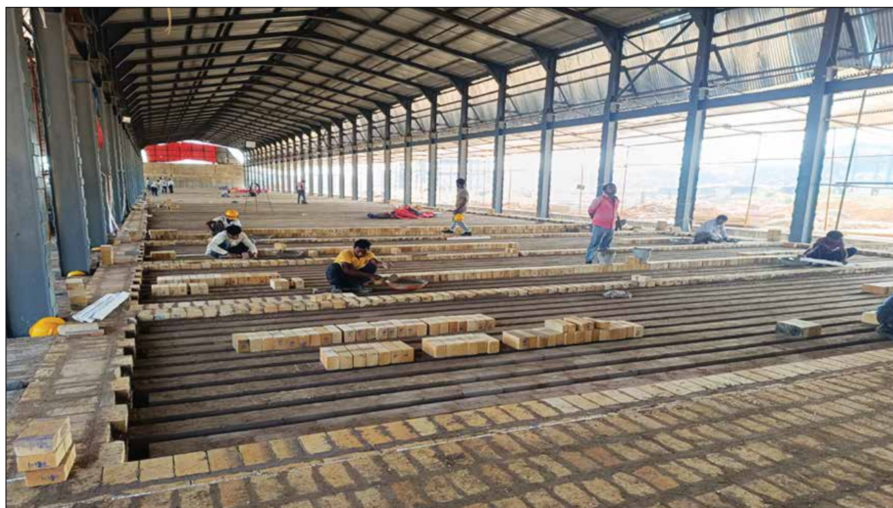
Refractory at Coke Oven Battery
